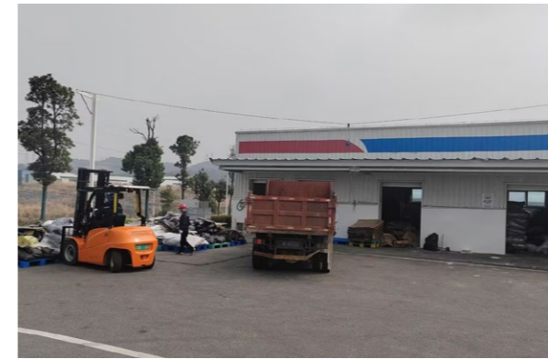
General Solid Waste Temporary Storage Area
