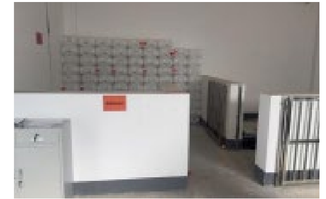
Hazardous Waste Storage Room
